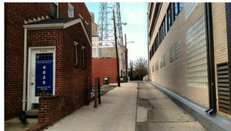
6. Alley view, looking north
