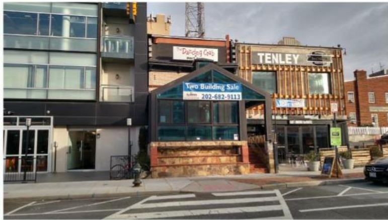
1. View of site from Wisconsin Ave, NW
