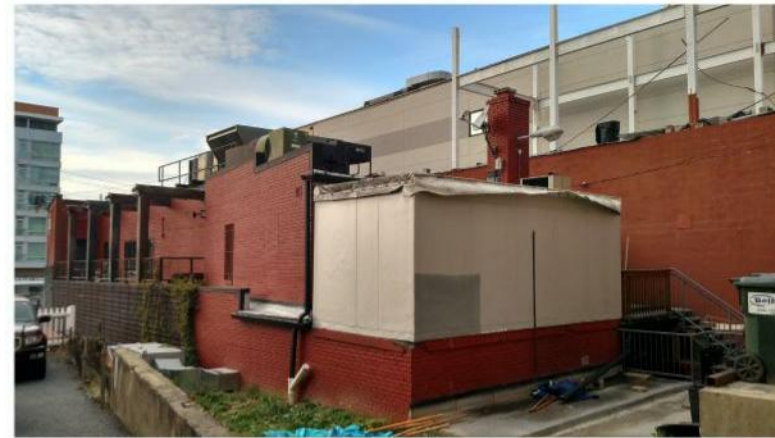
4. View from alley looking northwest
